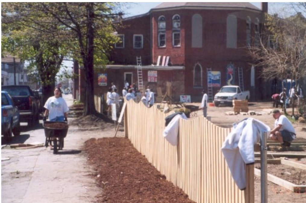
Potters Avenue Community Garden and Park — in progress
