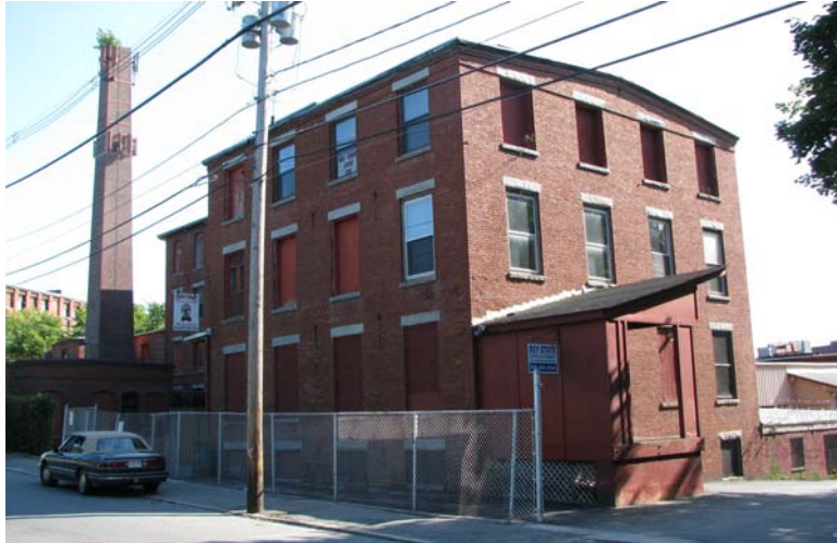
Erected in 1862 and located off Lawrence Street, Belvidere Woolen Mill No. 2 was expanded a number of times by the Stotts during the family's ownership of the company.
