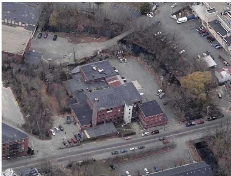
This aerial view shows the largely intact factory buildings of Belvidere Woolen Mill No. 2. Hale's Brook extends around the northern perimeter of the mill property which now contains a number of businesses.
